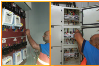
To troubleshoot & reinstall submeters at MRT stations - MRT Project (Bukit Bintang, Maluri, Jalan Bandar) -
