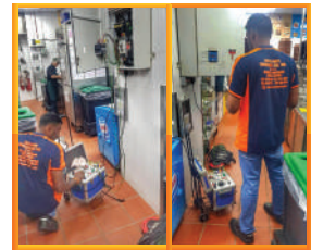
To Calibrate Protection Relays (IDMT & ELR) - Chilis Jaya
