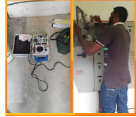
To replace 150A Terasaki Breaker, shunt trip coil & to calibrate IDMT - Masjid Nurul Ihsan, Taman Seri Cheras -
