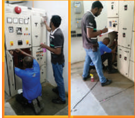
Testing, servicing of LV Switchgear, capacitor correction board and LV MSB panel - Batu Permai Apartments -
