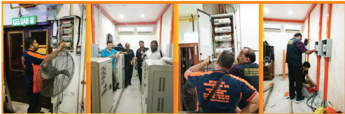
Installation of Automatic Voltage Stabilizers at Tioman Island.
